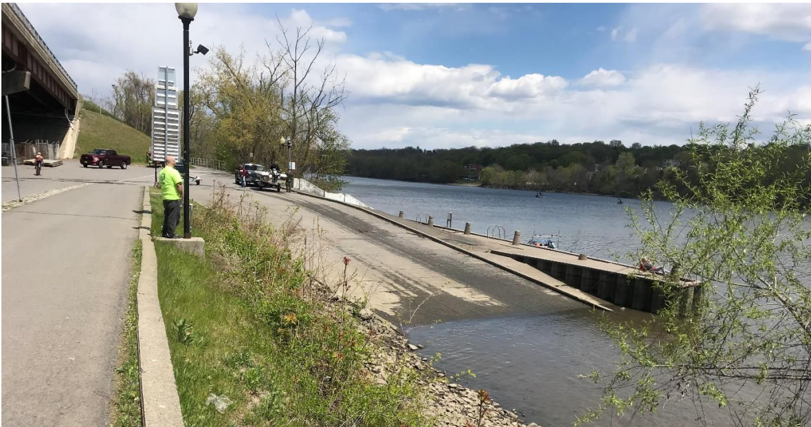
Figure 11: Existing Corning Riverfront Park boat launch.
