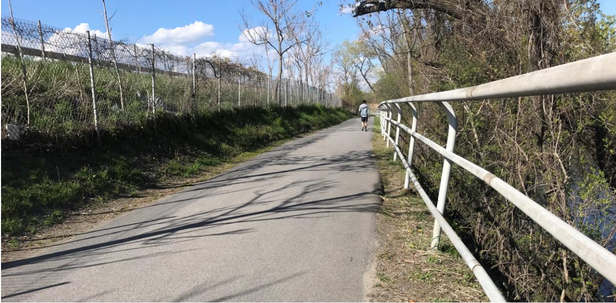
Figure 14: Pathway along I-787 at the Riverfront Preserve - the slope to the river is very steep
